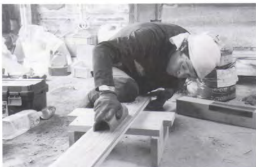
Adjusting convex roof tiles / 丸瓦調整
