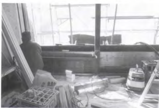
Restoration of the store, second floor 店舗 2 階修理
