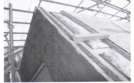
Restoring barge boards / 鉢巻
