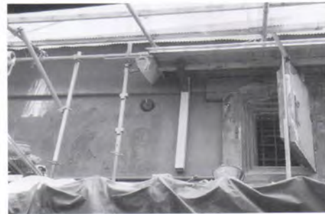
Application of brown coat, front façade 正面中塗り
