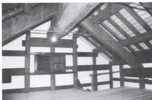
Third floor interior, after restoration / 3階修理後
