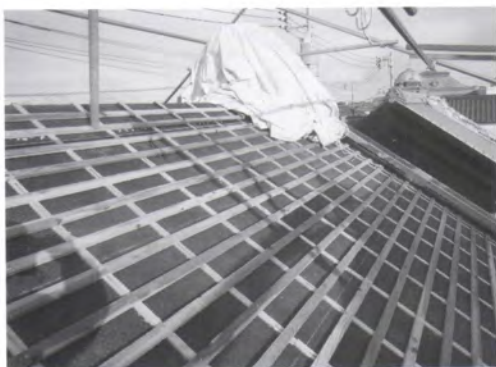
Preparing substrate for roof tiles / 瓦葺き下地
