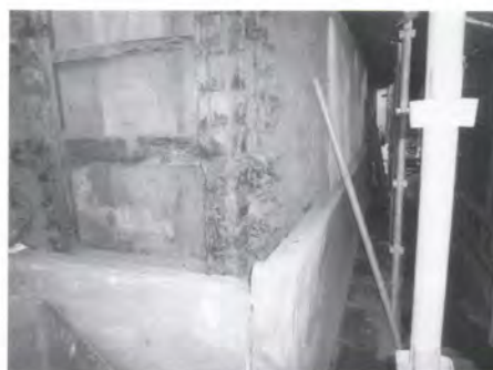
Storehouse, northwest corner 土蔵北西隅
