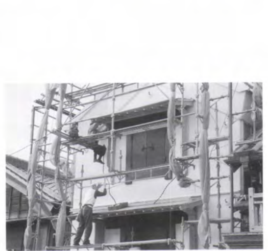
Plaster finish / 漆喰仕上げ
