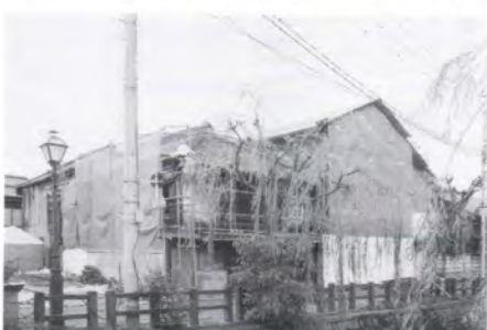
Roofted scaffolding / 素屋根
