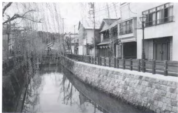
After restoration / 修復後
