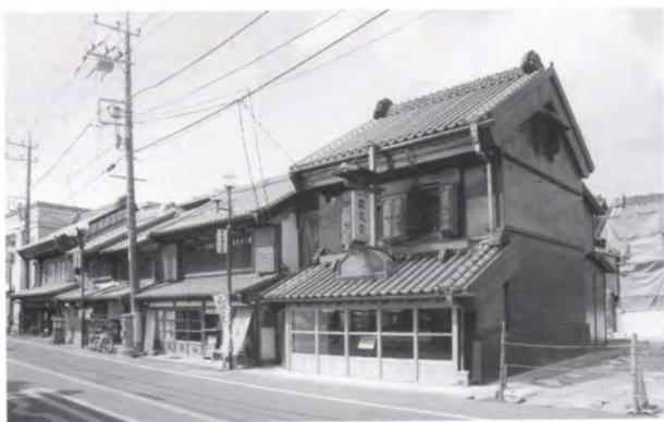
The revived streetscape of Sawara / 町並みが再生
