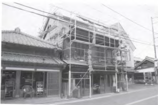
Scaffolding was built for restoration 修理用足場架け
