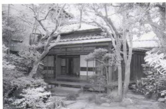
After restoration / 修理後
