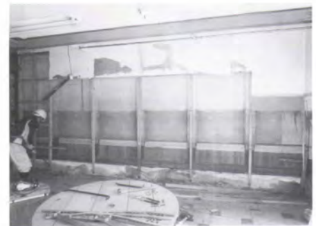
Repairing store interiors / 店舗内装修理
