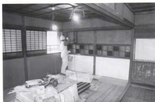
Applying mud on walls, third floor / 3階壁塗り
