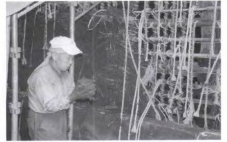
Applying mud on walls / 荒壁打ち
