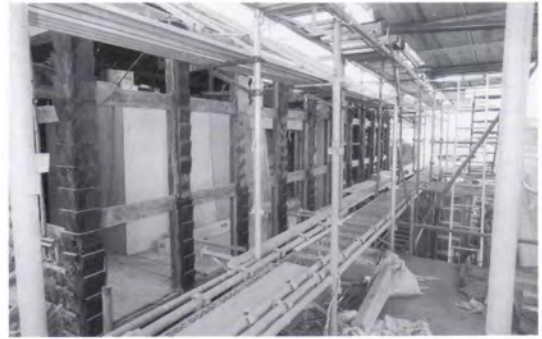
Removal of earthen-wall / 壁土を除去
