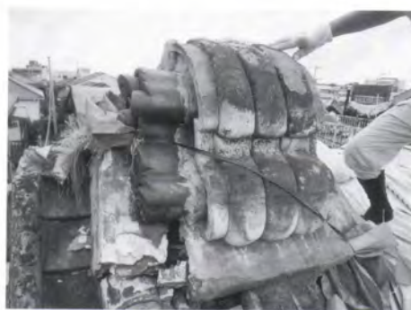
Plasterwork around ogre tiles 鬼瓦と影盛り
