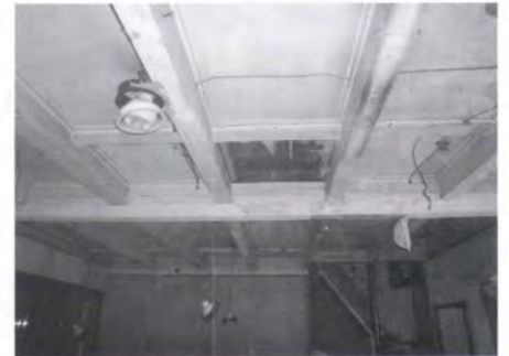
Repairs to store ceiling / 店舗天井修理
