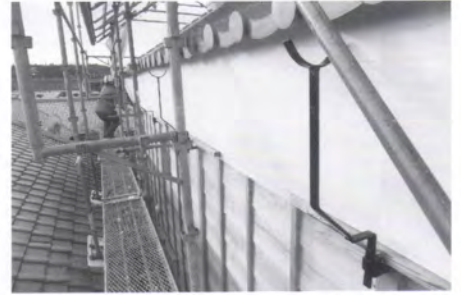
Plastered eave projection / 鉢巻
