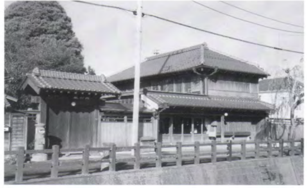
After restoration / 修復後
