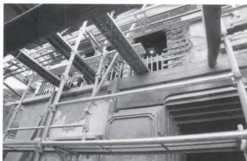
Storehouse, front façade repairs / 土蔵正面修理
