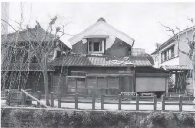
Right after the earthquake / 被災直後
