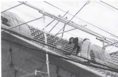
Main ridge / 棟積み
