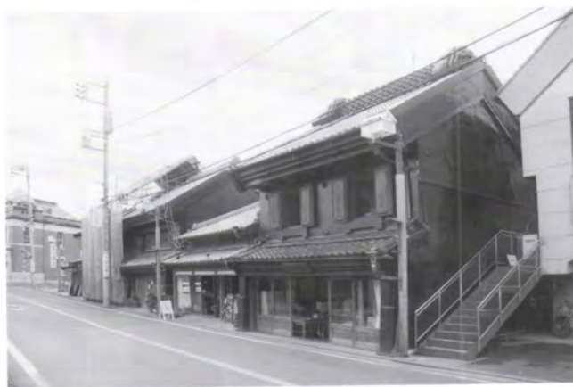
After restoration / 修理後
