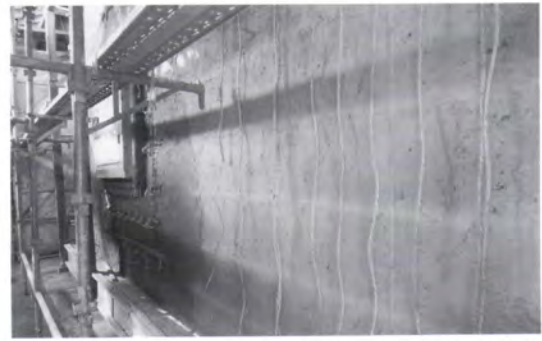
Application of brown coat / 中塗り
