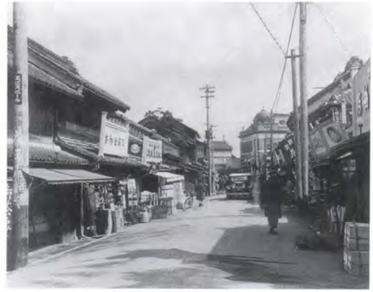
Looking east from Chukei-bashi Bridge 忠敬橋から東方
