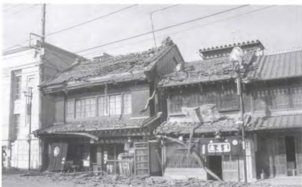
Right after the earthquake / 被災直後
