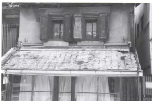
Roof substrate of front eave / 下屋庇下地
