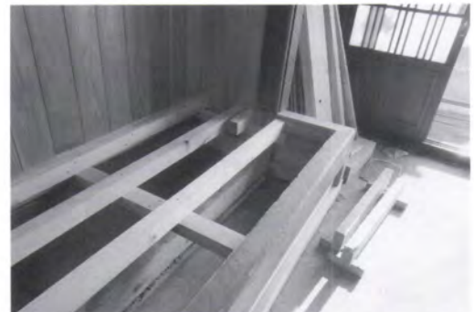
Restoration of tatami-matted floor, first floor 座敷復元修理
