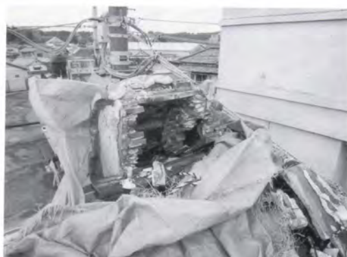
Plasterwork around ogre tiles / 影盛り
