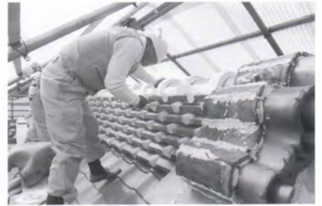
Plastering the main ridge / 棟積み
