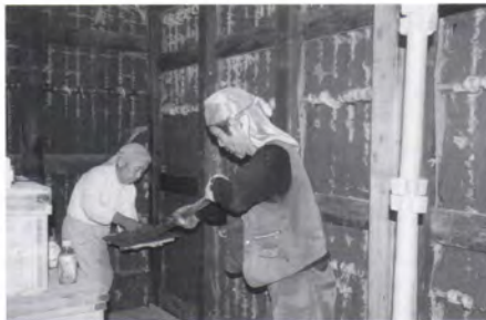
Applying mud on opposite sides of walls 荒壁の裏打ち
