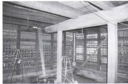
Weaving the bamboo lattice substrate 小舞掻き
