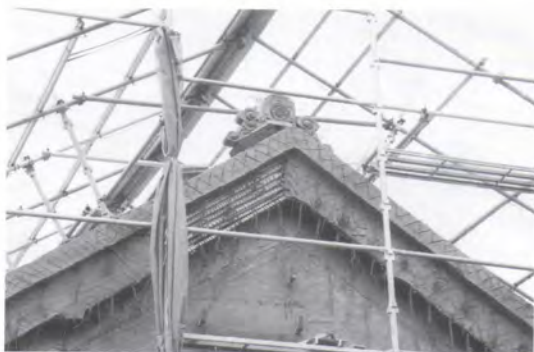
Repairing the storehouse gable / けらば修理
