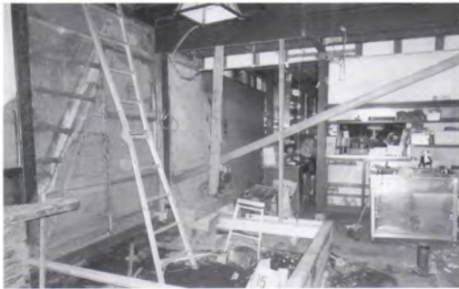
Repairs on foundation and walls / 基礎・壁修理
