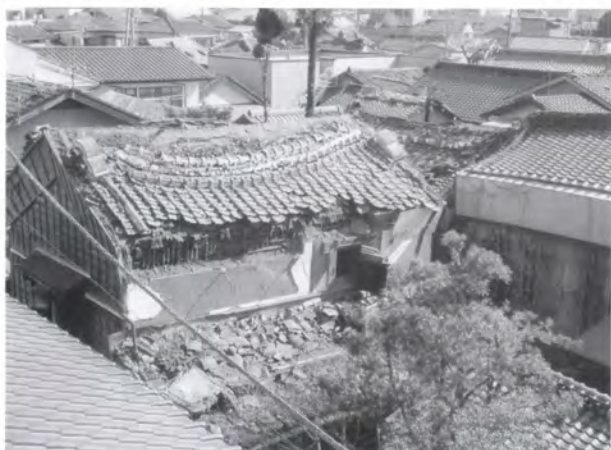
Right after the earthquake / 被災直後
