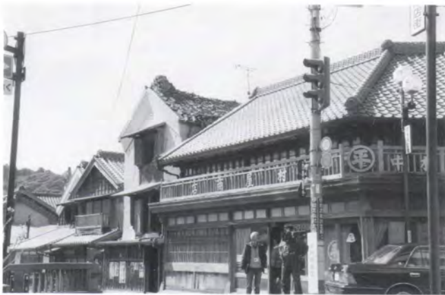
Right after the earthquake / 被災直後
