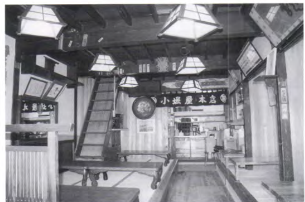
Store interior, after restoration / 修理後
