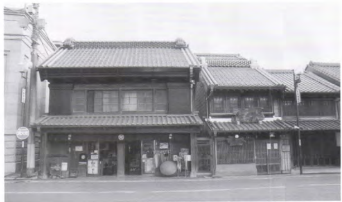
After restoration / 修理後
