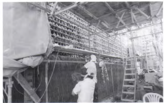
Wall substrate and application of mud 小舞と荒壁打ち
