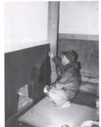
Plaster finish on lower walls 腰巻仕上げ
