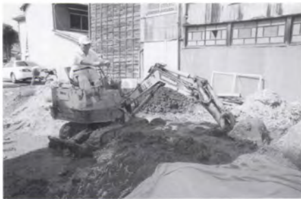
Preparing mud for walls / 壁土捏ね
