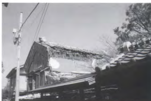
Storehouse, view from north / 土蔵北側
