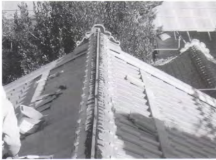
Main ridge of store annex / 平屋棟積み
