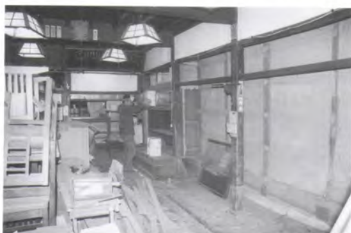
Restoration of the store, east wall 店舗東側面修理
