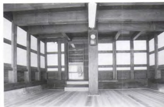
First floor store, after restoration / 1階店舗修理後
